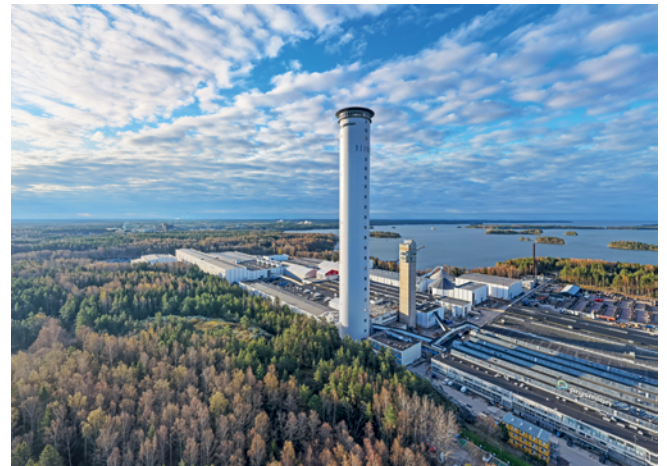
18 Prysmian Sky Project
