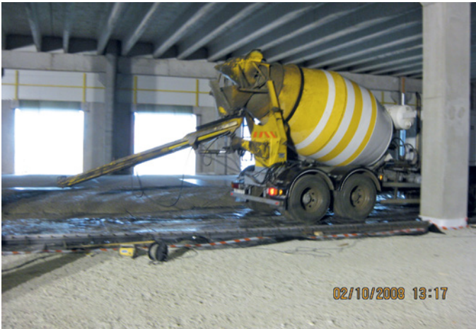
5 Lattian valua betoniautosta
