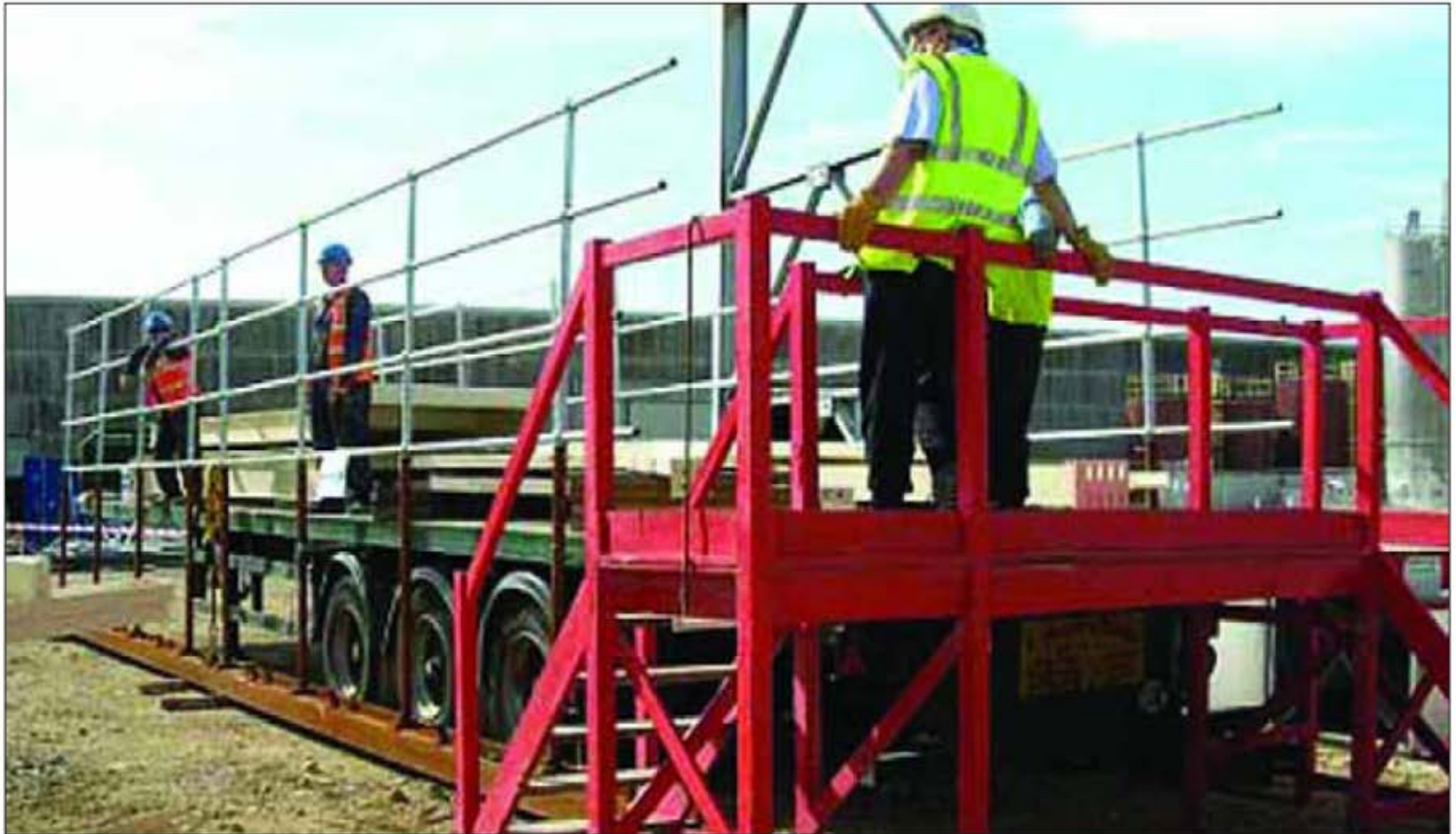
Figure 1 Trailer edge protection system with access platform and steps
