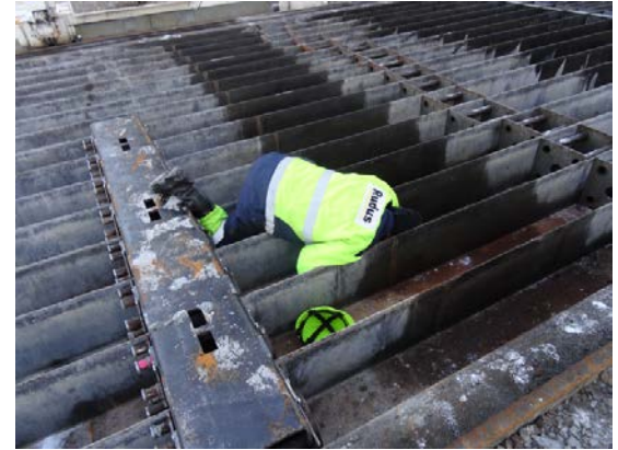
Place where accident happened notice slippery stopper
