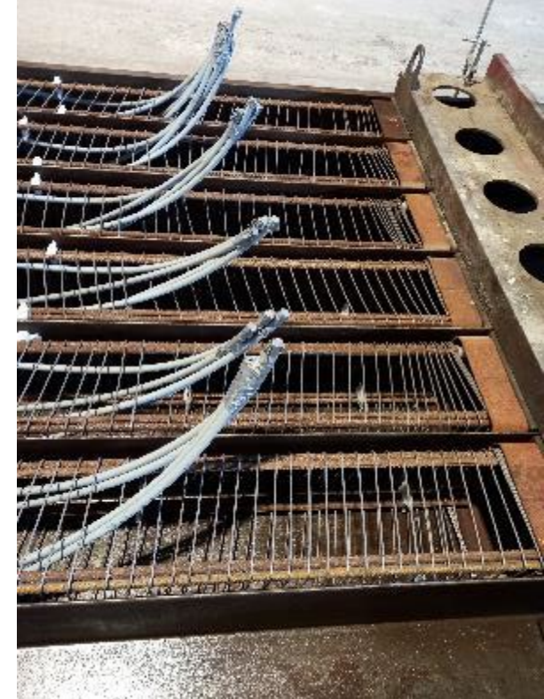
Pipes coming out of pile head
