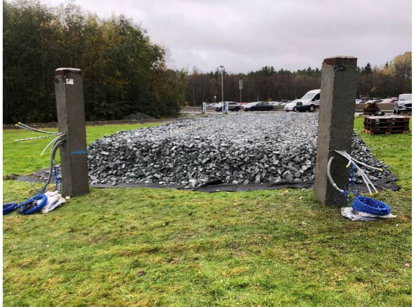
Two Driven Energy piles were successfully installed on 16 th and 17 th October 2023
