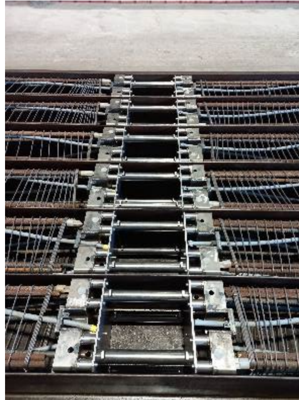
Joints and Casting guides are installed
