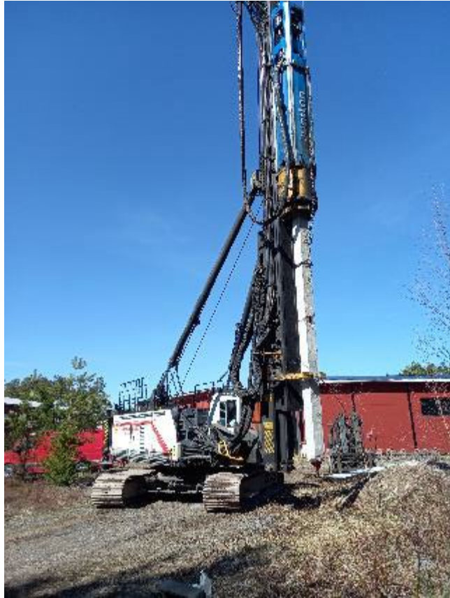
Moving the piles to the test box
