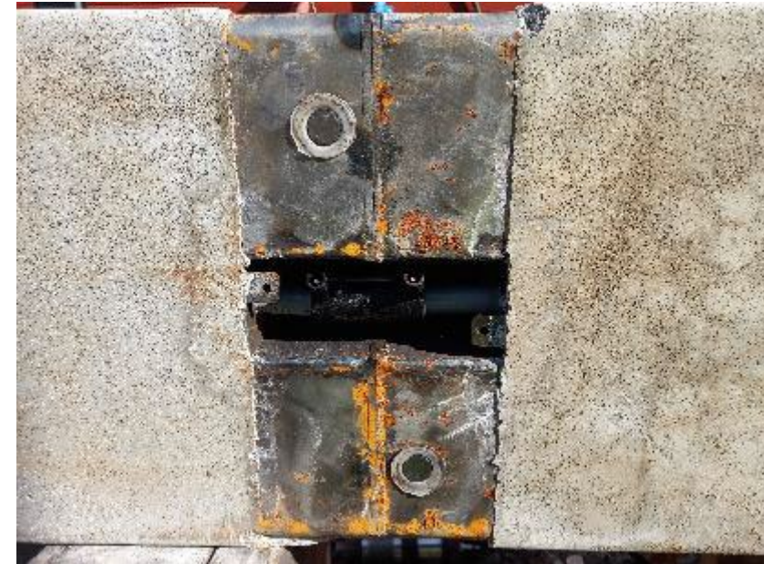
Pins installed, and pipe fittings connect the pipes
