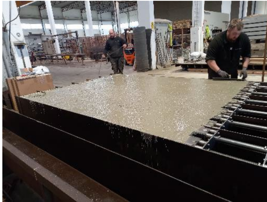
Finishing the surface
