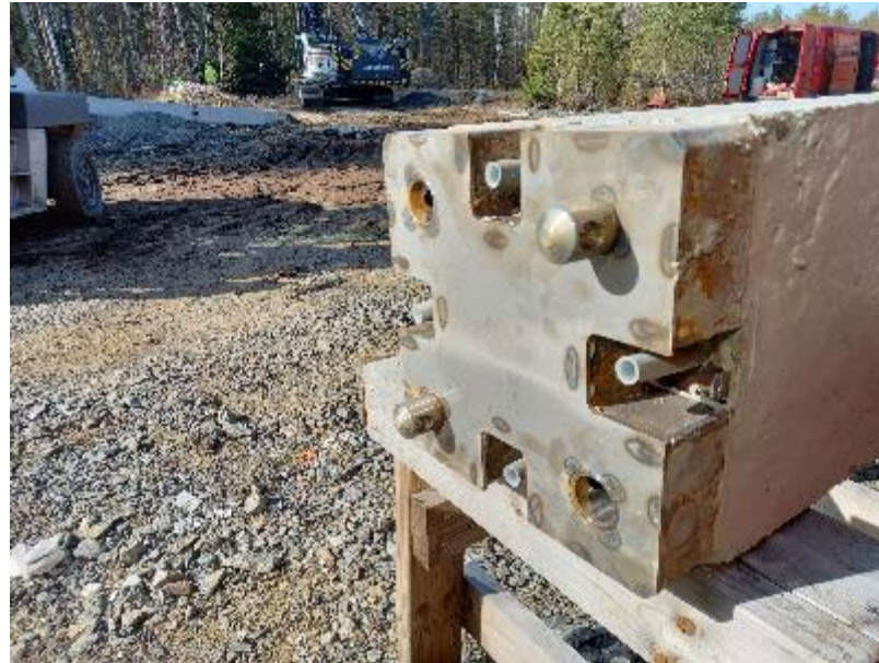
Preparing the pipes
