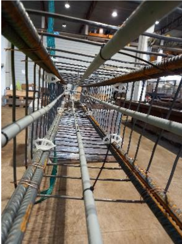
Installation of Pipes in the cage
