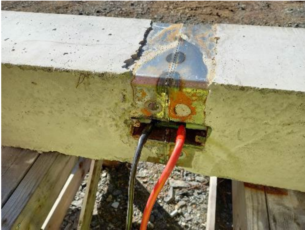
25 second welding + 5 min cooling time
