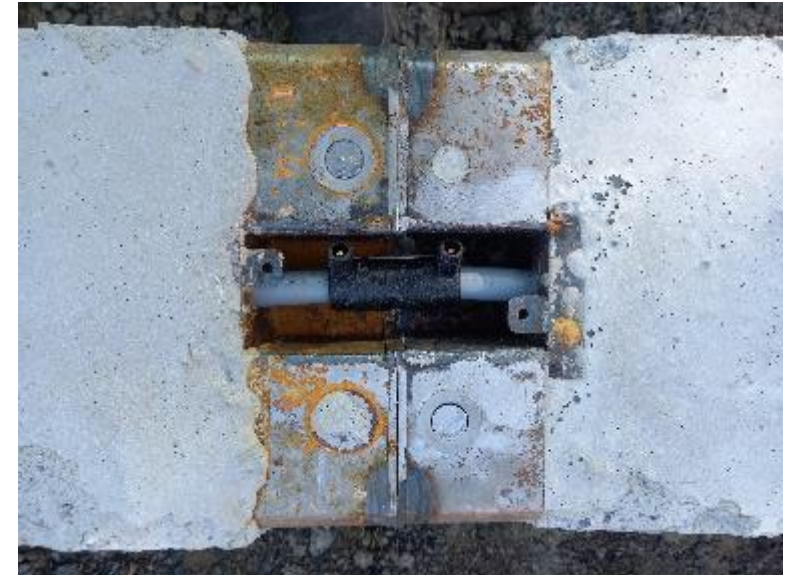
No leakage observed and pressure drop is less than 5%
