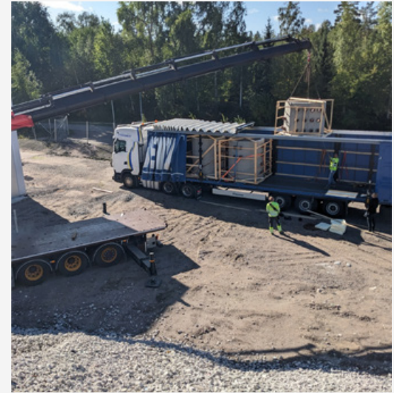
The lifting operation was performed outside of Hyperion's facility
