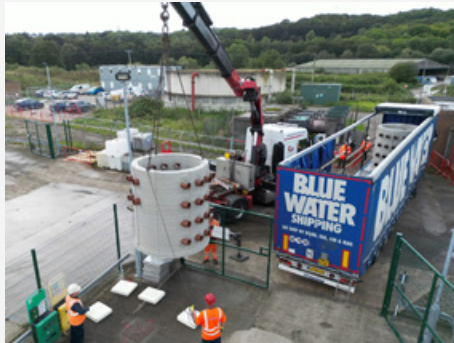
MMB's team inspecting the drawpits
