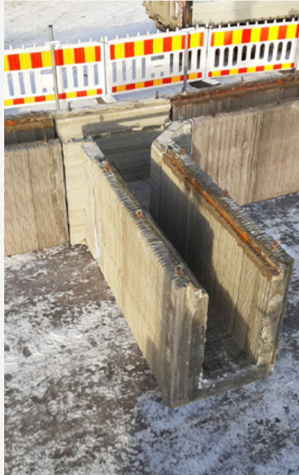
Trenches and Nodes
