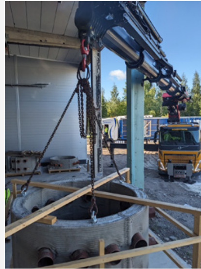
View from the top of the lifting arrangement.
