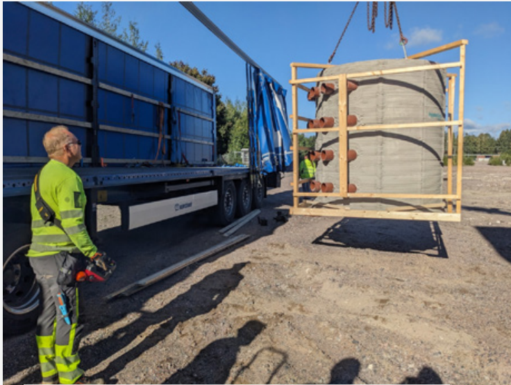
Driver of the crane positioning the drawpits near the flatbed truck
