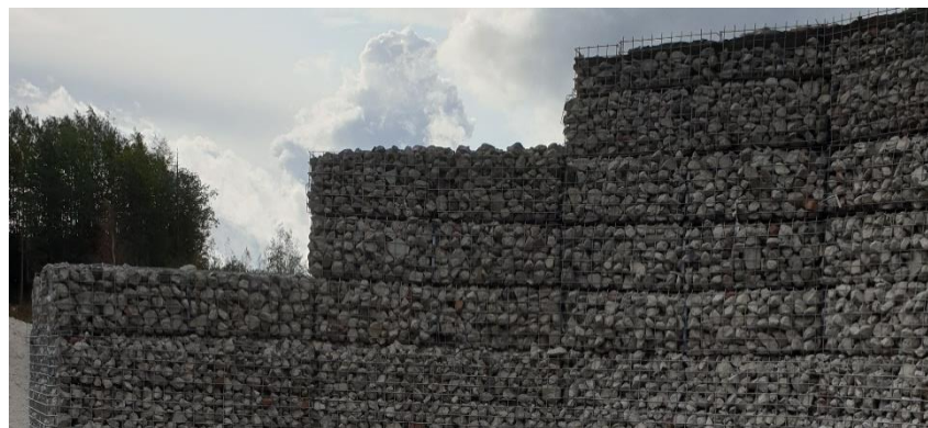
Picture 1: A sound barrier made of recycled concrete rocks at a recycling plant of Rudus.
