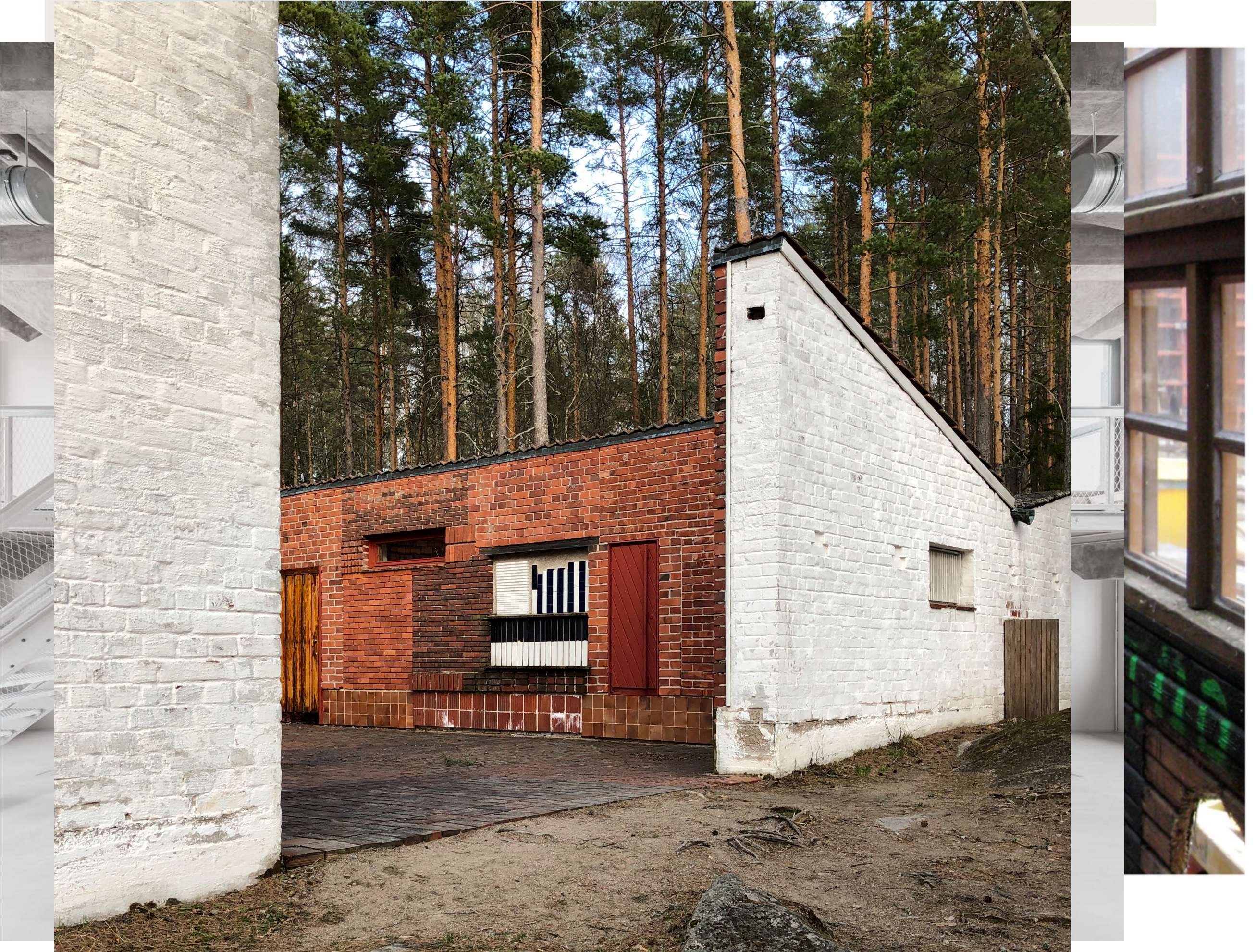
Alvar Aalto: Muuratsalo Experimental House; 1952-54
